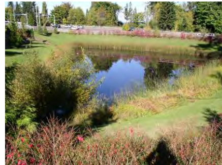
Figure 49. Example of regional storm water pond.
