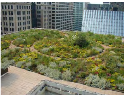
Figure 48. Green roof, Chicago, IL.
