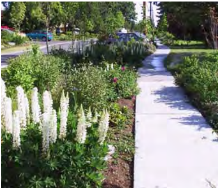
Figure 46. SEASStreet vegetated bioretention swale. Seattle, WA.
